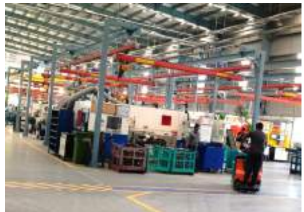
XY RAILS (STEEL) WITH HOIST
